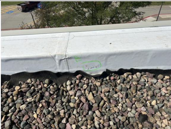
Install target patch at damaged membrane.
