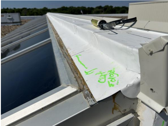
Clean and prime Aluminum before membrane. Install cut edge sealant on reinforced membrane.
