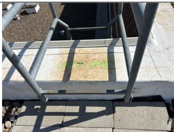
Install walk pad on membrane at ladder top.
