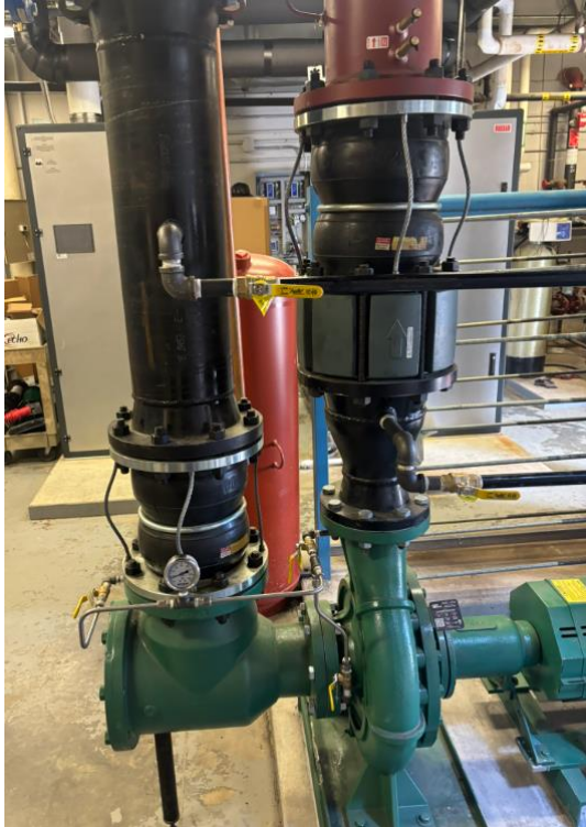
Photo 5: No strainer present in pump headers.
