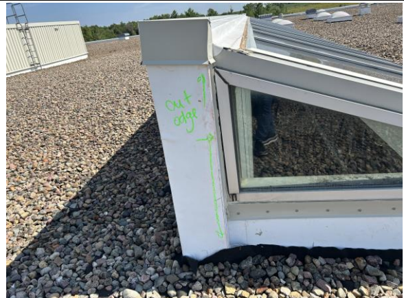
Cut edge sealant required.
