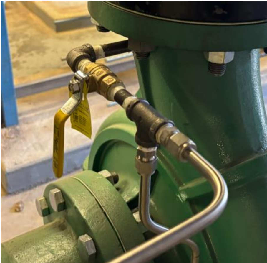
Photo 8: Black steel pipe installed for pressure differential piping on pumps.
