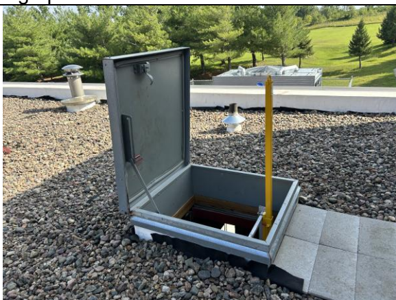
Install hatch railing when delivered.
