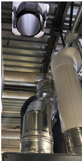
Photo 10: Boiler exhaust ductwork not connected.
