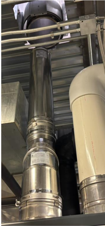
Photo 9: Boiler exhaust ductwork not connected.
