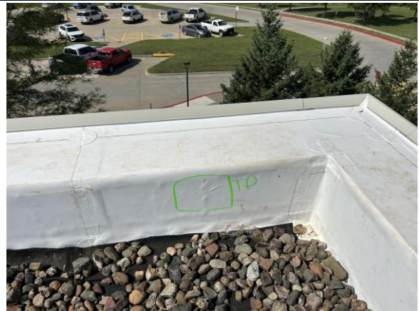
Install target patch at damaged membrane.
