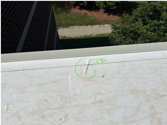
Install target patch at creased membrane.
