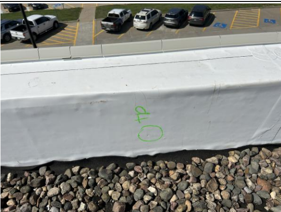
Install target patch at damaged membrane.
