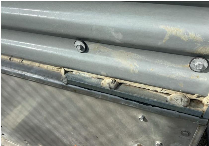
Photo 6: Cooling tower gasketing has water leaking through.
