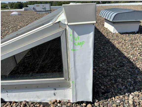
Cut edge sealant required.
