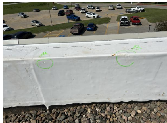
Install target patch at damaged membrane.
