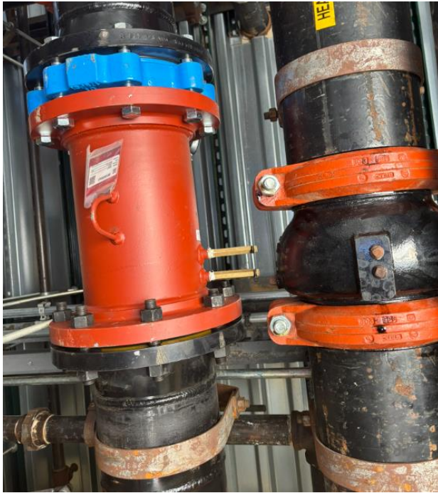
Photo 3: New balancing valve ports not accessible.
