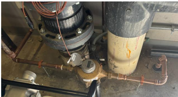
Photo 1: Broken gauge.
