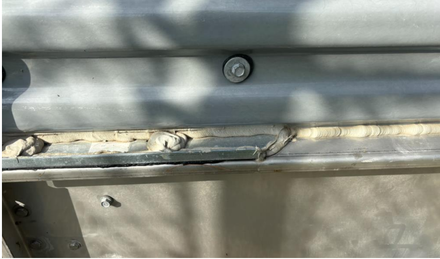
Photo 7: Cooling tower gasketing has water leaking through.
