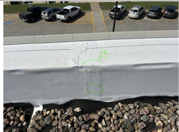
Install target patch at damaged membrane.
