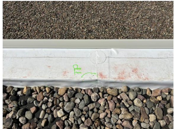
Install target patch at damaged membrane.
