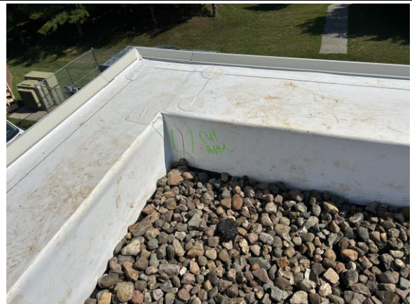
Install cut edge sealant at cut reinf. membrane.
