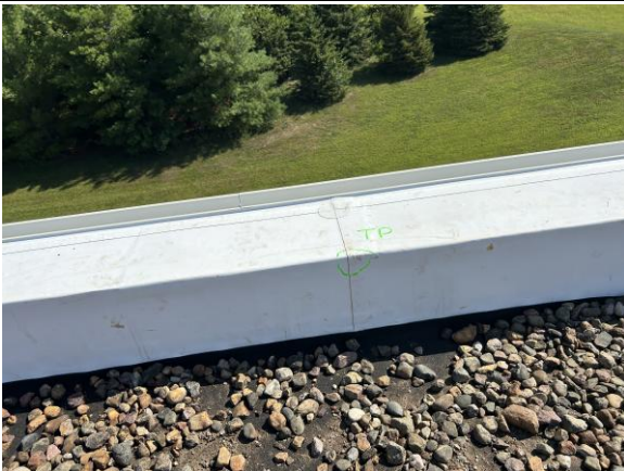
Install target patch at damaged membrane.
